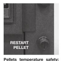
In the rare event there is a too high temperature in the tank, the thermostat for pellets safety with manual reset creates an alarm "FLAR-SIC-FAIL" stopping the pellet boiler stove. You need to reset the system working on the device placed on the back of the thermostove.
